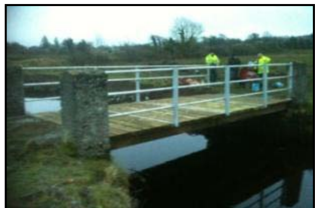
Steward’s Bridge - After’
