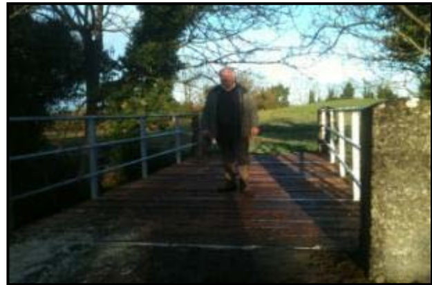
‘Haverty’s Bridge - After’
