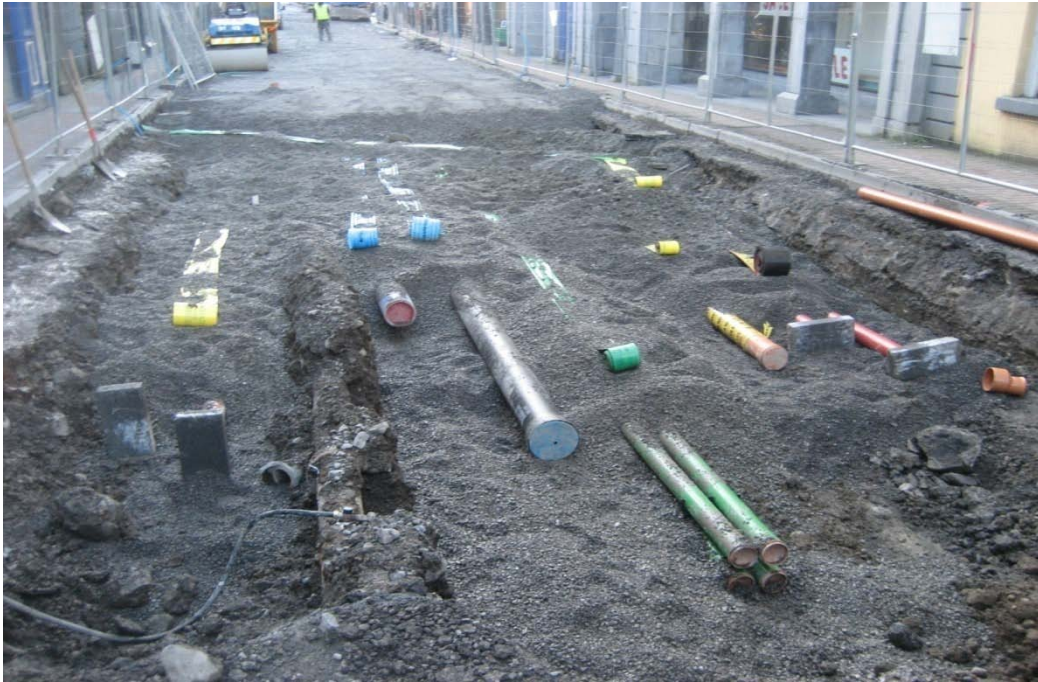
Both pictures above showing excavations along Bishop Street.
