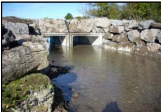
L-8555 at Caherawoneen South – After
